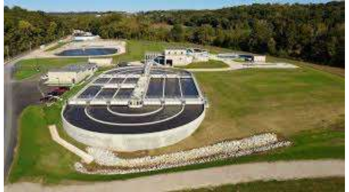
Medium scale aerobic wastewater treatment facility
