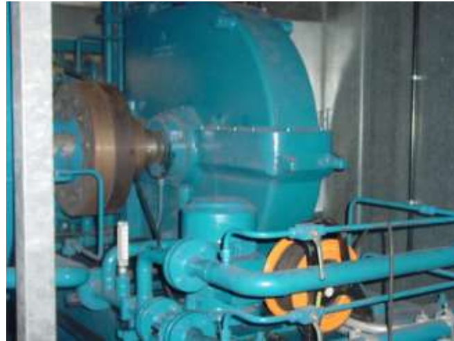
Back pressure turbine in action
